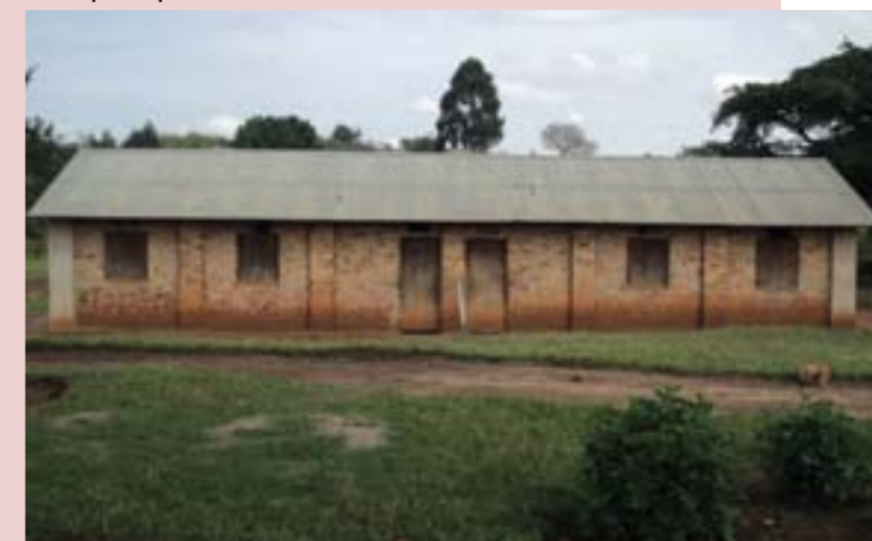
A two classroom block at Mpara primary school put up by parents but left incomplete due to inadequate capacity.
